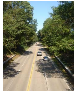
The parkway retains its historic character with four lanes. Photo by G. Booth
