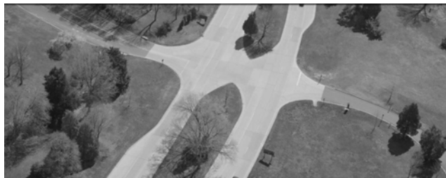
A concern of the original design of the parkway is at-grade crossings and limited sight-lines. Photo by NPS
