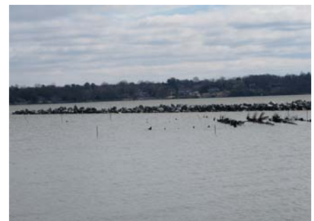
The breakwater extends 1,500 feet into the marsh. Photo by Glenda Booth
